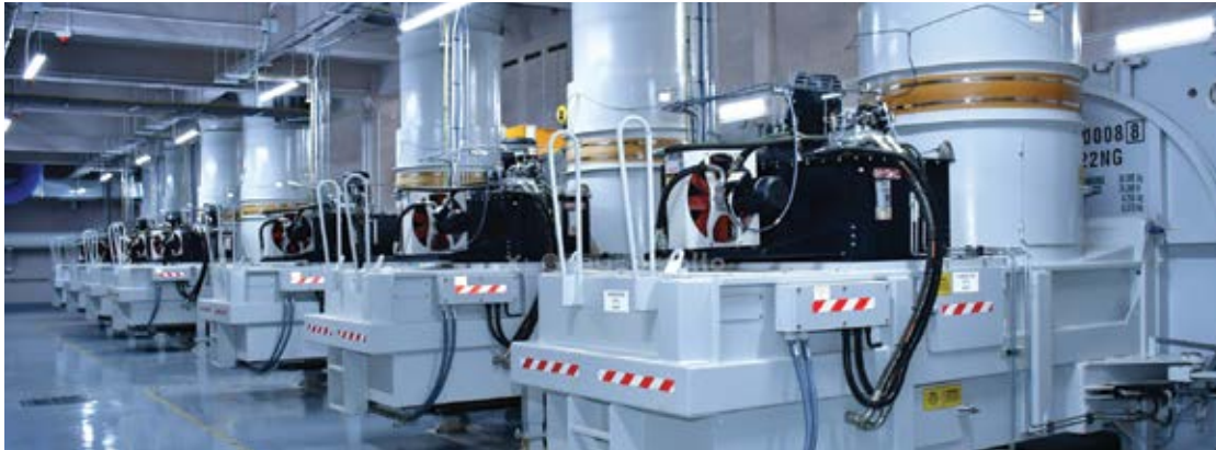
The continent's first automated pneumatic solid waste management located at the Konza Technopolis.
