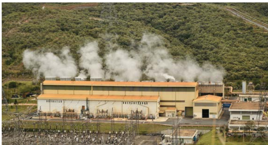
One of the geothermal generating power plant at Olkaria area of Naivasha where Kenya Generating Electricity Company (KenGen) has established an over 8,000-acre green energy park where investors will access direct and lower power tariffs, relaxed customs and tax reliefs. PHOTO: ERASTUS GICHOHI
